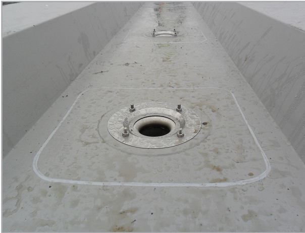
Good installation, prior to siphonic outlet inlets being installed
