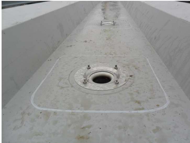
Good installation, prior to siphonic outlet inlets being installed
